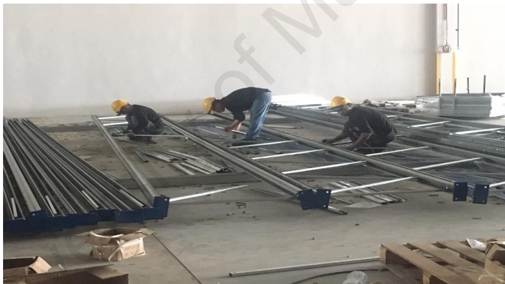
Figure 4-4 Frame Assembly Process
