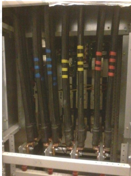
(a) Cable used as an outgoing from switchgear
