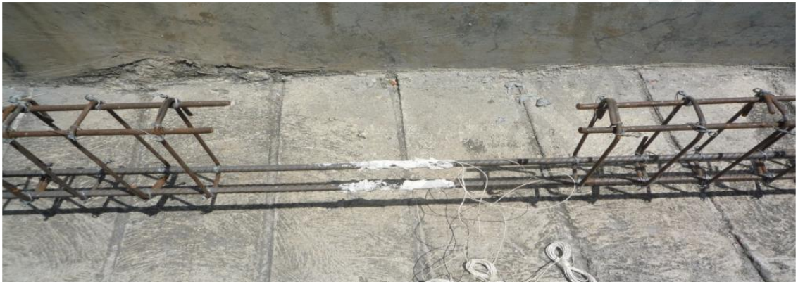
Figure 3.13: Strain gauges covered with silicone gel
