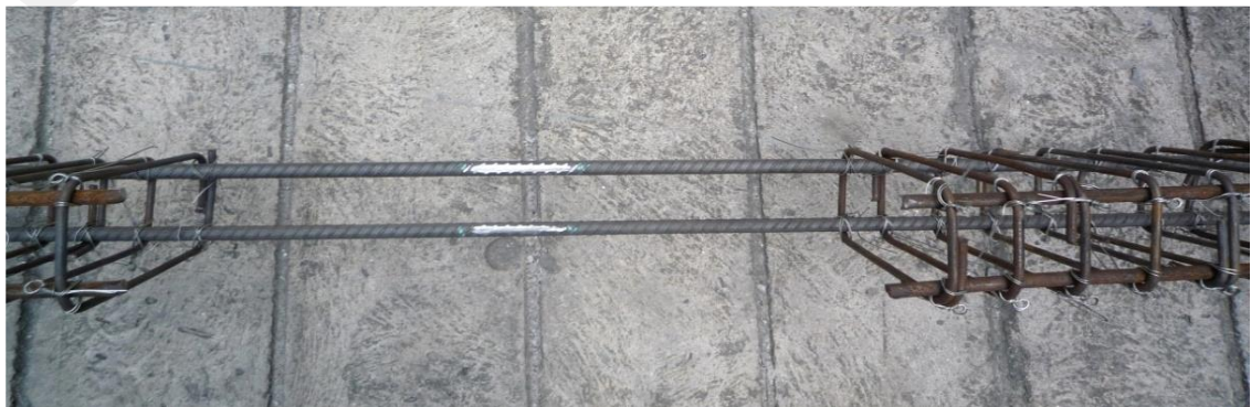
Figure 3.12: Surface preparation of steel bars to place strain gauges
