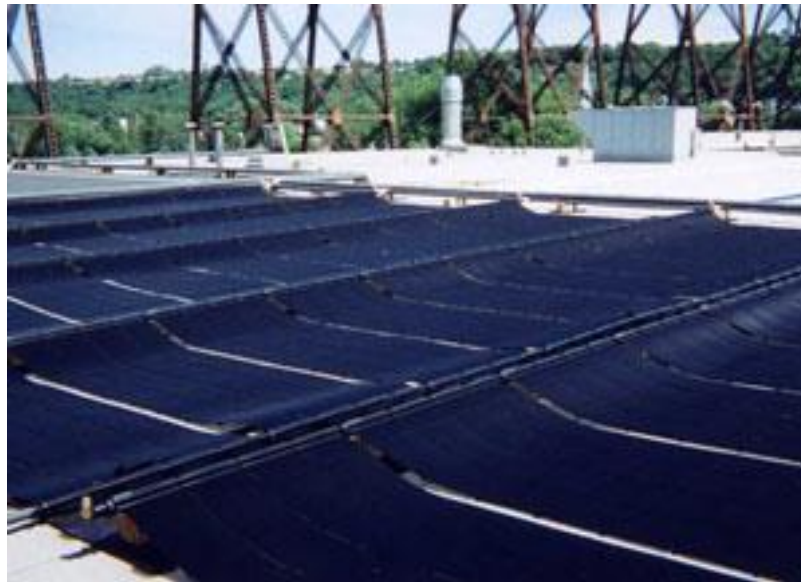
Figure 2.2 Unglazed flat-plate collectors (RETScreen, 2011).
