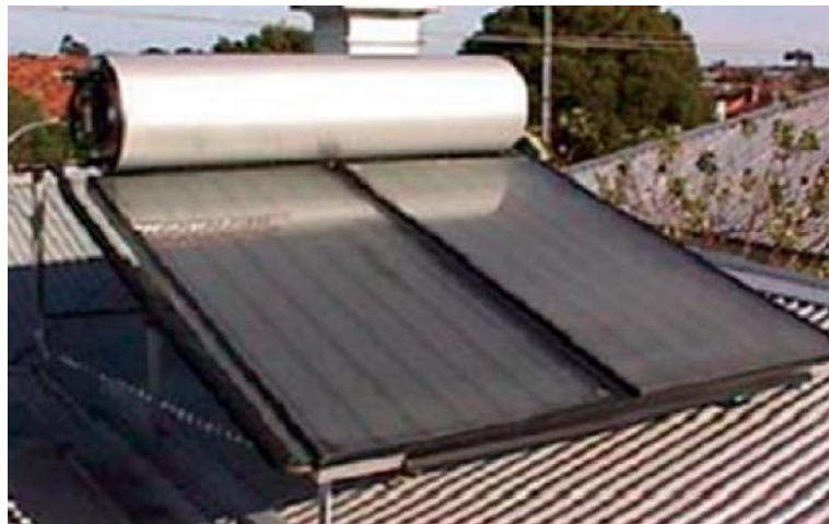
Figure 2.7 Solar Domestic Hot Water (Thermosiphon) Systems in Australia.
