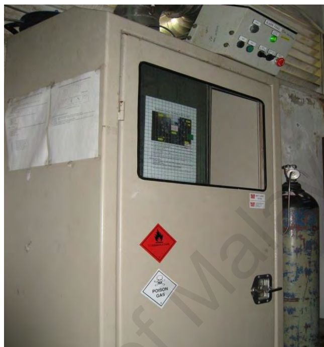
Figure 3.9: Silane Gas Control System.
