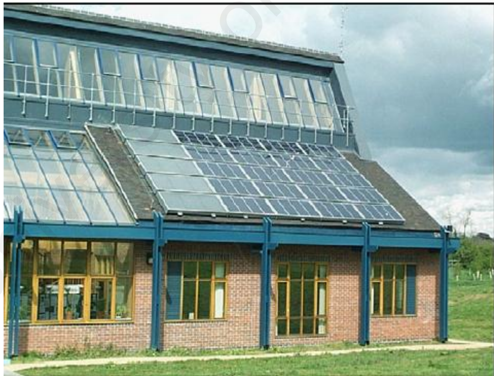
Figure 2.10: PVT system mounted on The Brockshill Environment Centre (Cartmell et al., 2004)
