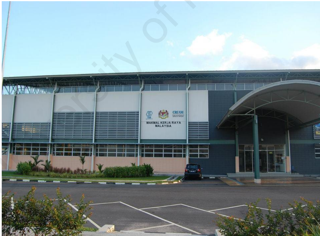
Figure 5.1: CREAM building, Kuala Lumpur
