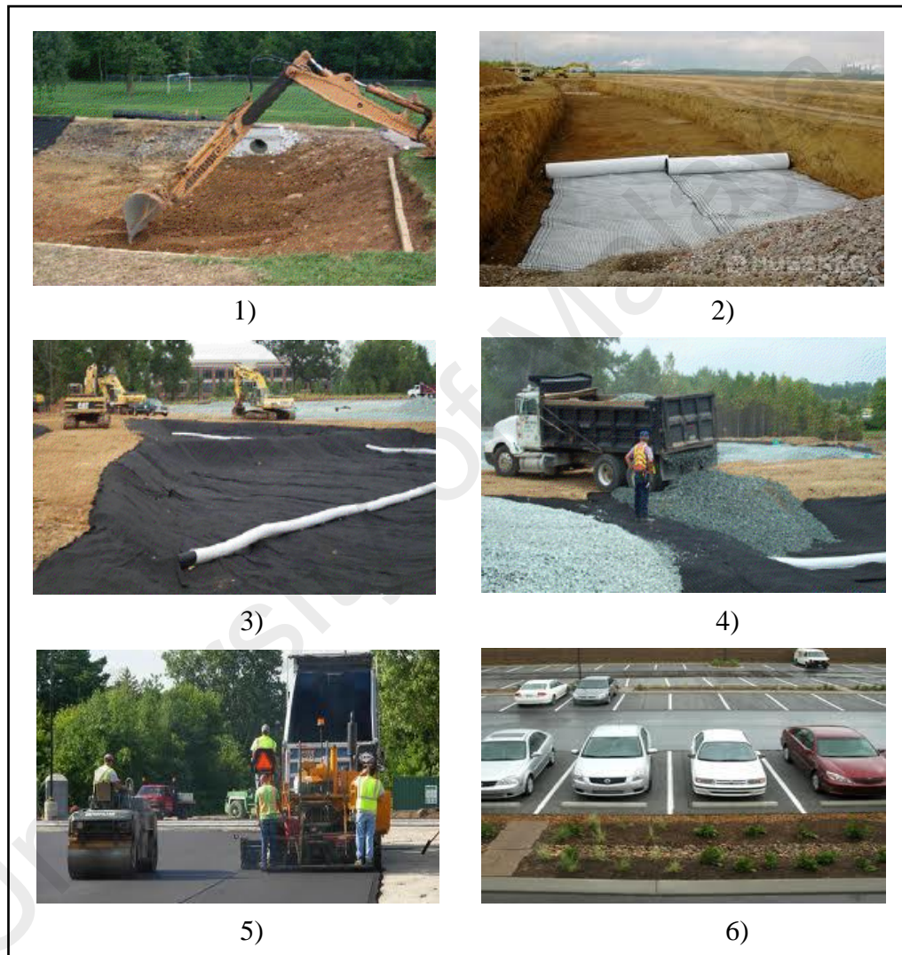
Figure 2.3 Sequence of Porous Asphalt Installation
