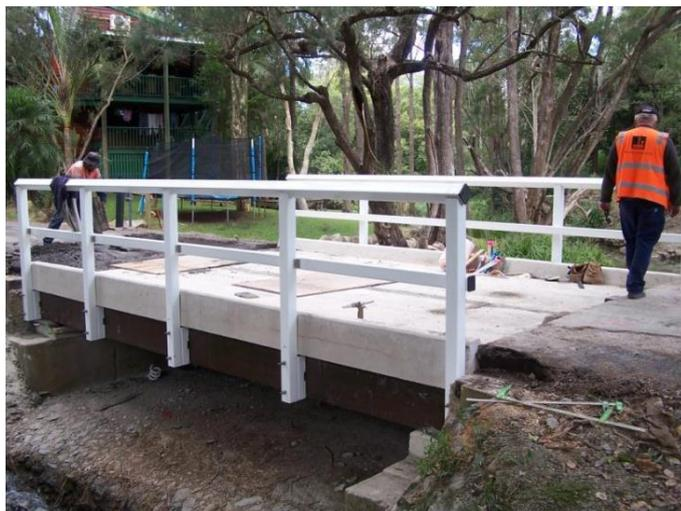
Figure 2.7: Composite pultruded girder and Grade 40 geopolymer deck bridge in Brisbane (Aldred & Day, 2012)
