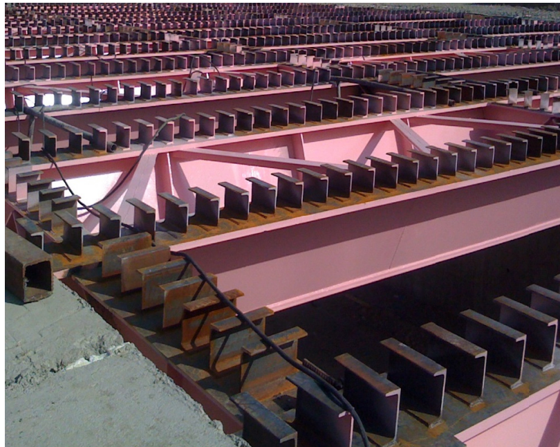
b) C-shaped channel shear connector
