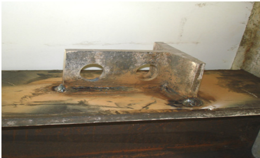
Figure 2.3. T-Rib shear connector
