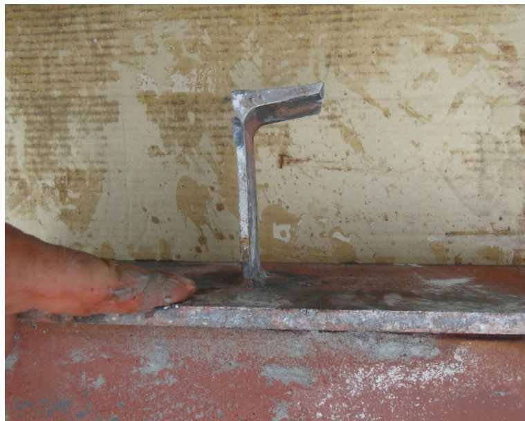
Figure 2.5. Typical angle shear connector
