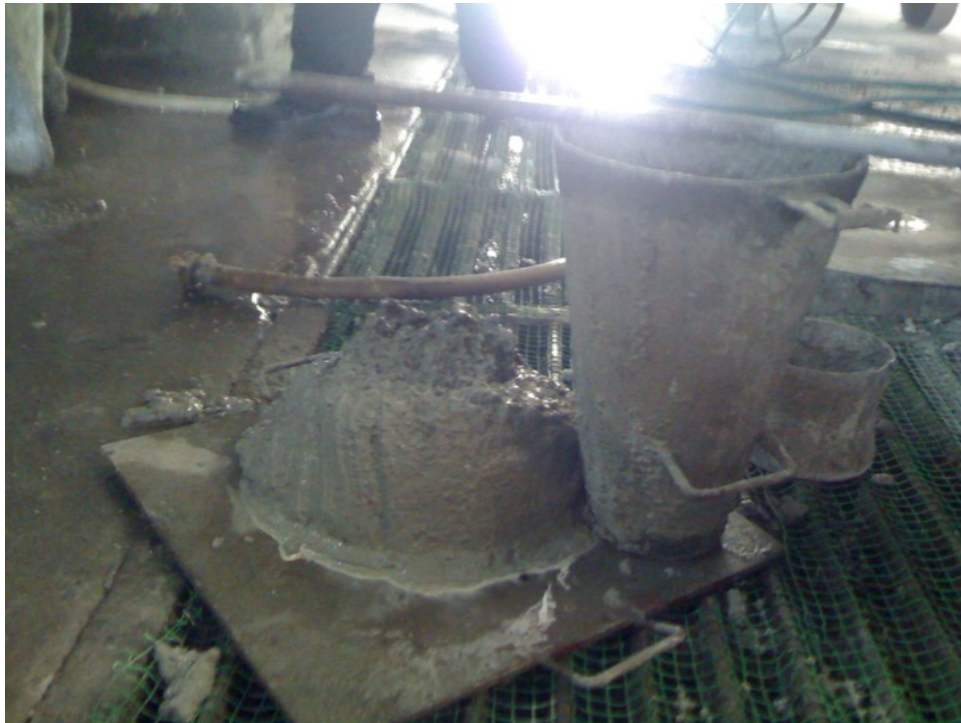
Figure. A.2. Slump test for concrete
