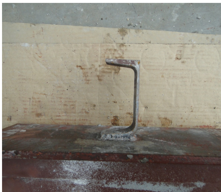
Figure 2.6. Typical channel shear connector
