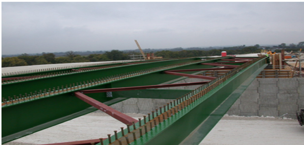
Figure 2.1. Headed stud shear connector
