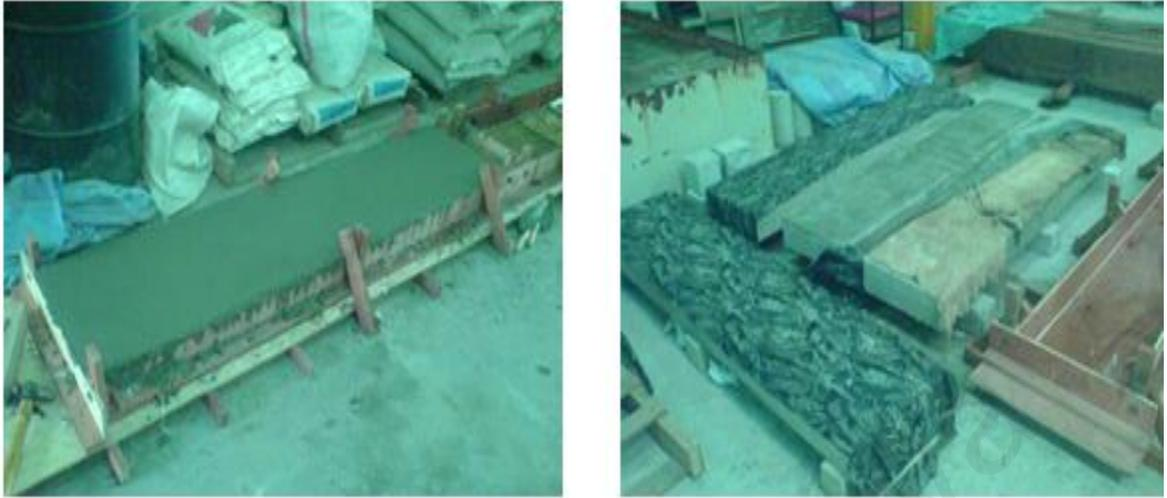
Figure 6.4: The casting and curing of the slabs
