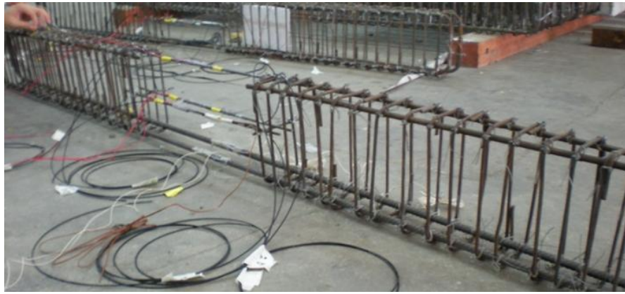
(a) Photograph of reinforcement for full-scale reinforced CB.
