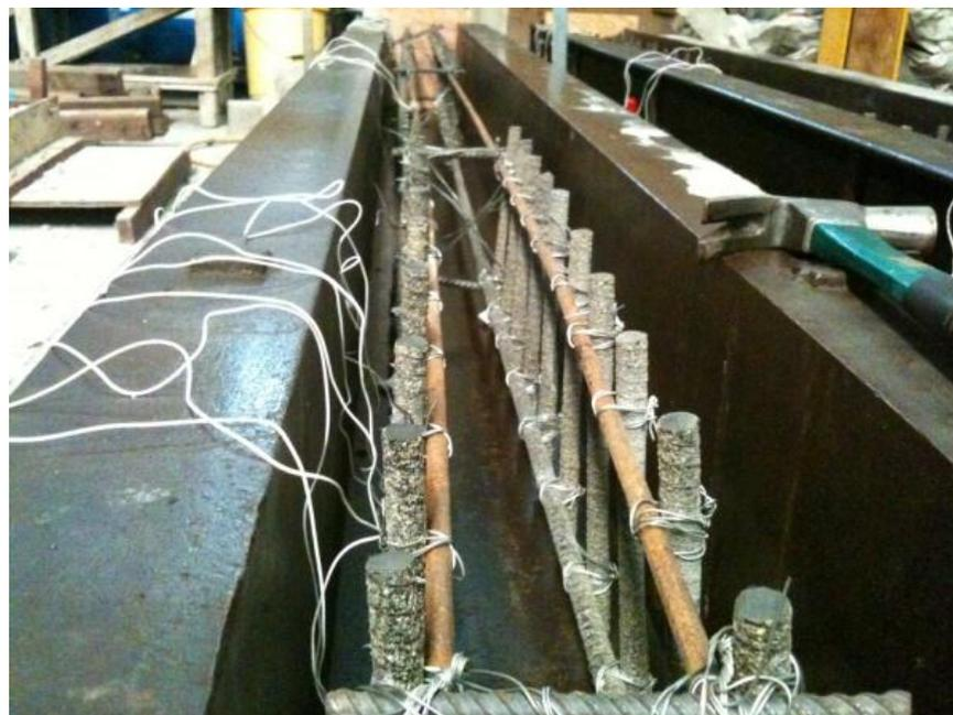
Figure 4.5.2 Group-I beams in moulds to cast -  $B_2C_{12}C_{12}@10$
