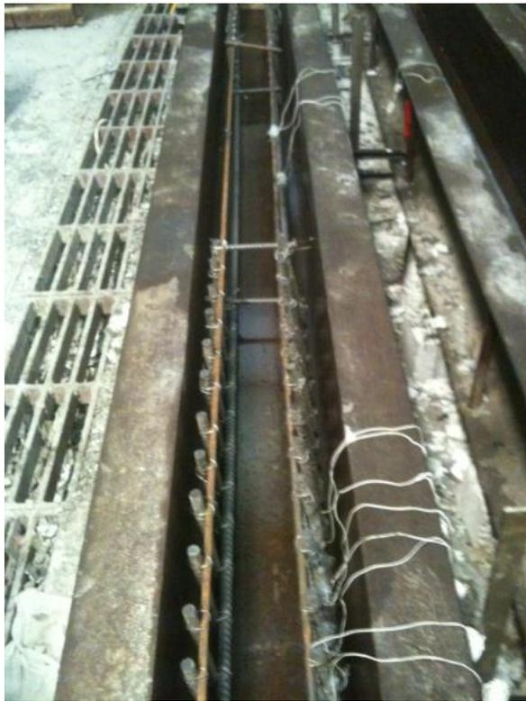
Figure 4.7.3 Group-II beams in moulds to cast -  $B_7S_{14}C_{12@7}$
