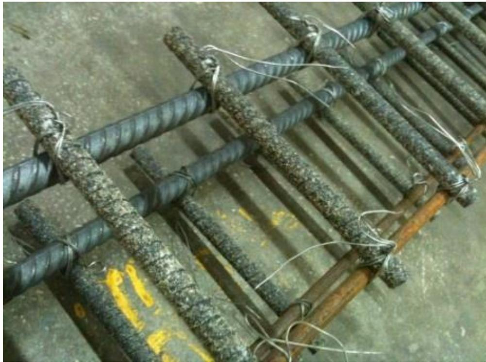
Figure 4.8.2 Installation and setup of shear reinforcement bars
