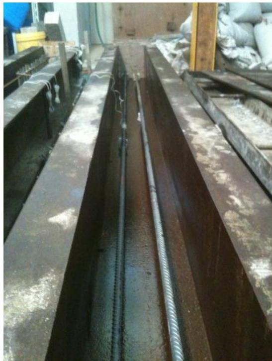
Figure 4.7.2 Group-II beams in moulds to cast -  $B_6S_{14}$
