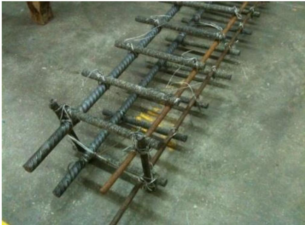
Figure 4.8.3 Installation and setup of shear reinforcement bars
