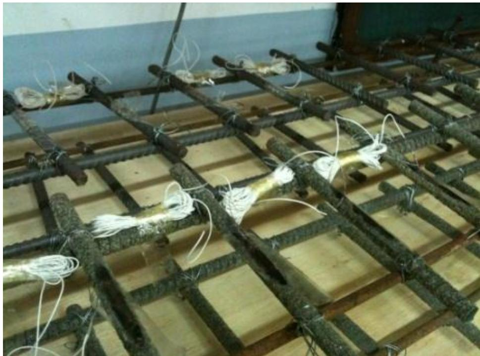
Figure 4.8.1 Installation and setup of shear reinforcement bars
