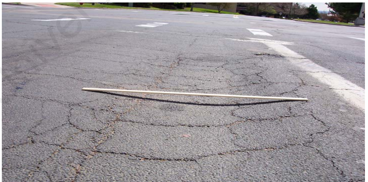
Figure 2.5 Permanent Deformations (Rutting)
