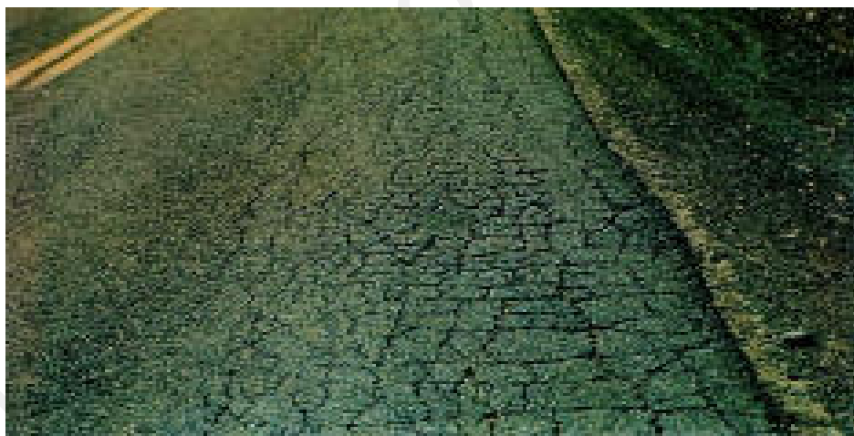
Figure 2.8 Fatigue Cracking
