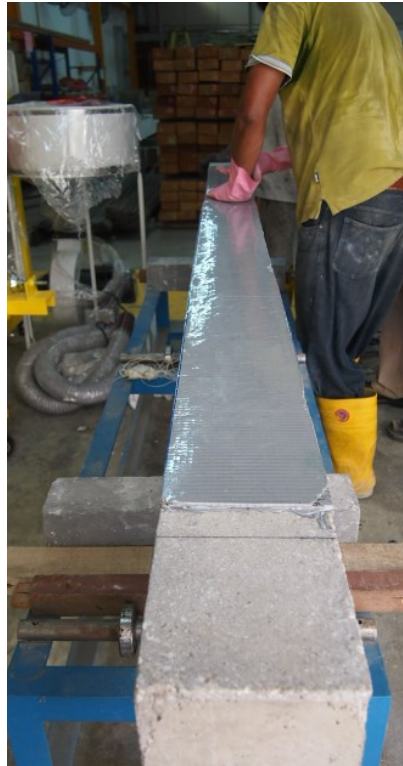
Figure 3.13: Placement of the wire mesh-epoxy laminate on beam surface
