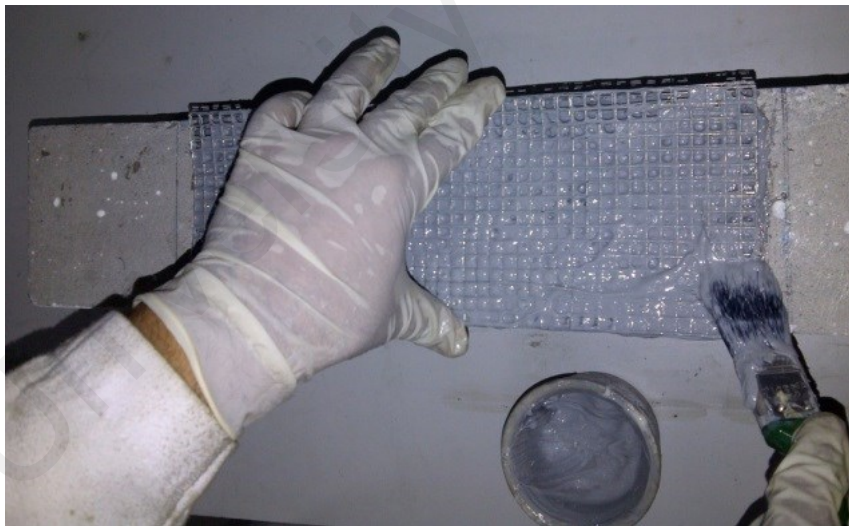
Figure 3.6: Applying of epoxy on multiple layers of wire mesh
