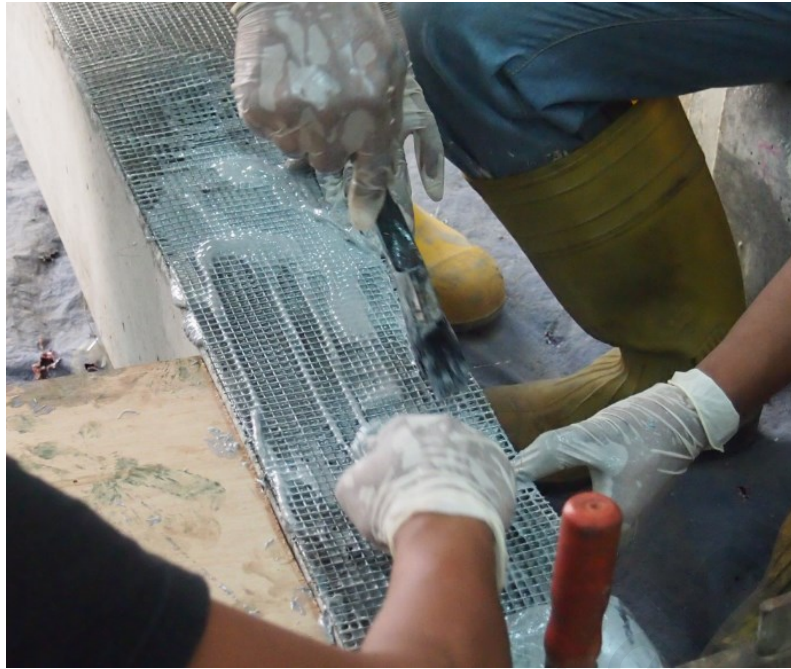
Figure 3.11: Applying epoxy on multiple layers of wire mesh placed on beam surface
