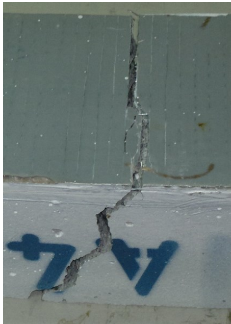
Figure 4.5: Failure of wire mesh-epoxy composite in specimen A4
