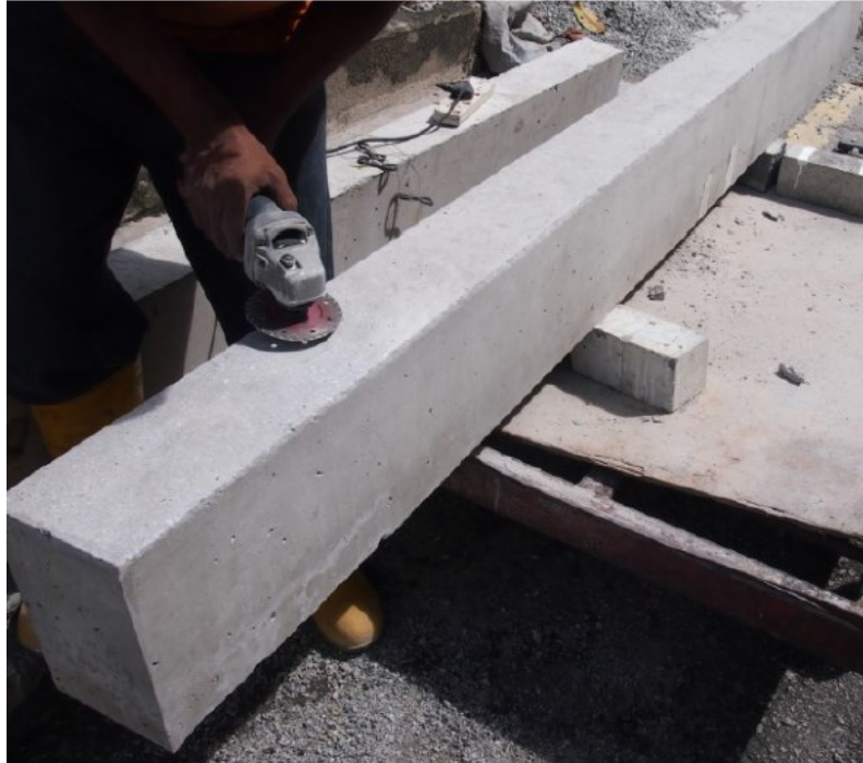
Figure 3.9: Surface preparation of RC beam
