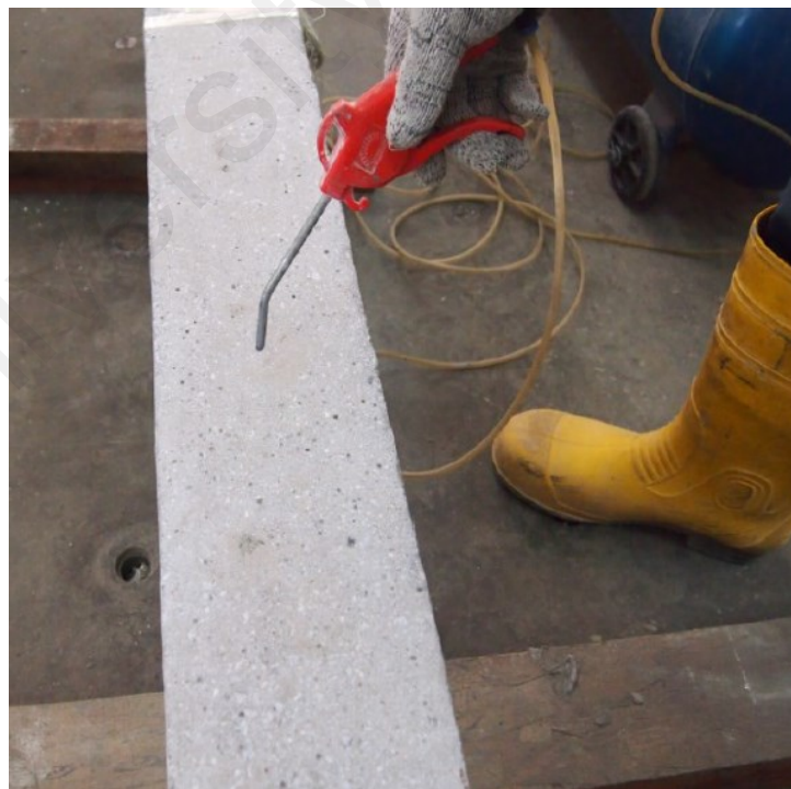
Figure 3.10: Removing of dust and loose materials by vacuum air cleaner
