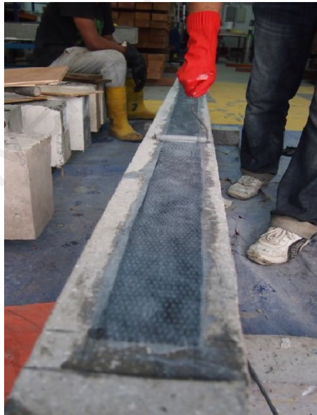
Figure 3.14: Strengthening of beam with CFRP sheet
