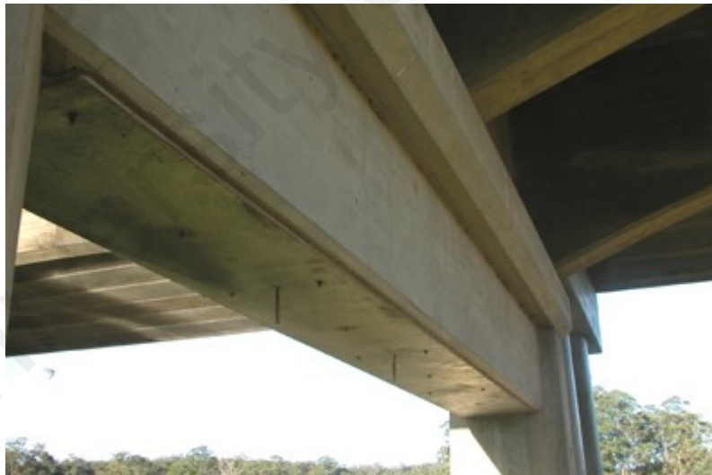
Figure 2.2: RC bridge strengthened using steel plate (Roads & Maritime- New South Wales, 2014)
