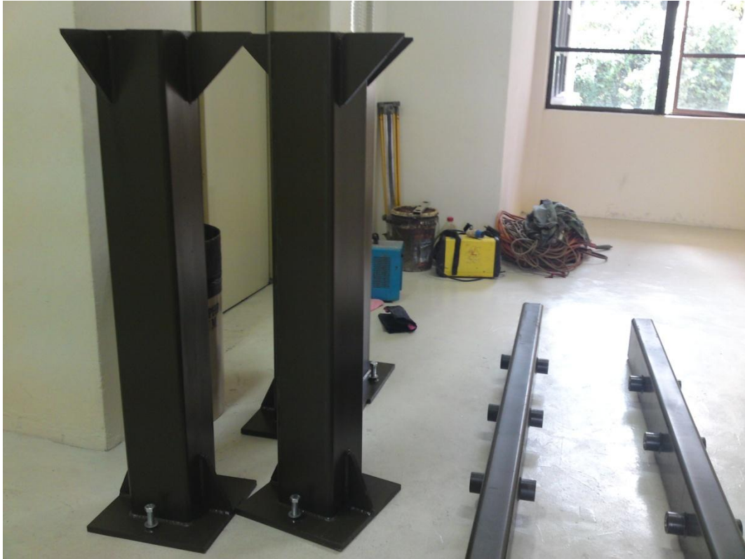
Figure 5.3: Steel columns to support the frame.
