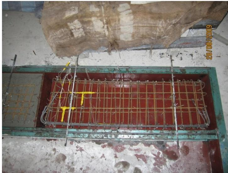
Figure 3.6: Casting arrangement of deep beam
