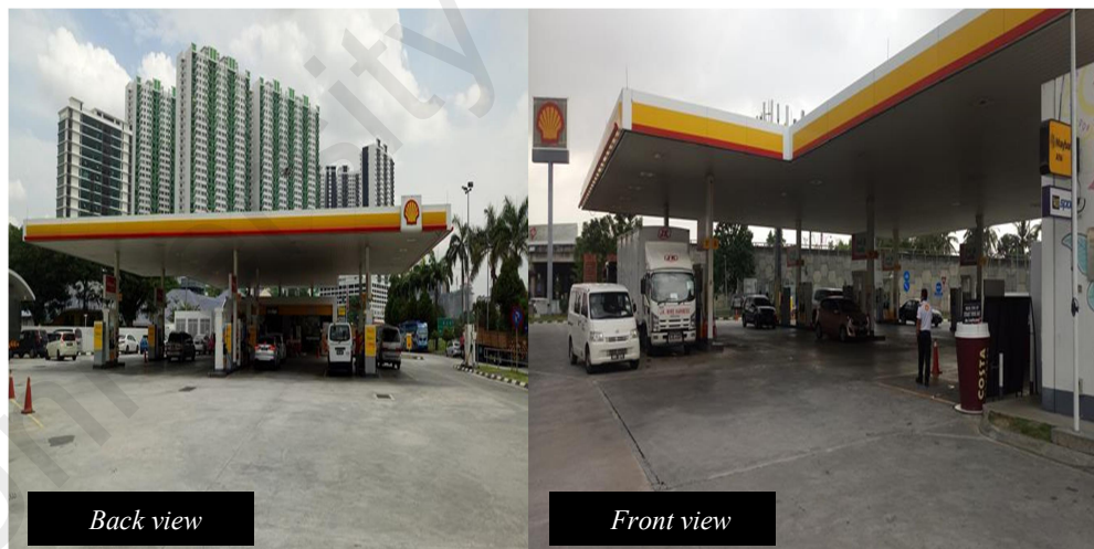
Figure 4.2 Forecourt area of the petrol station
