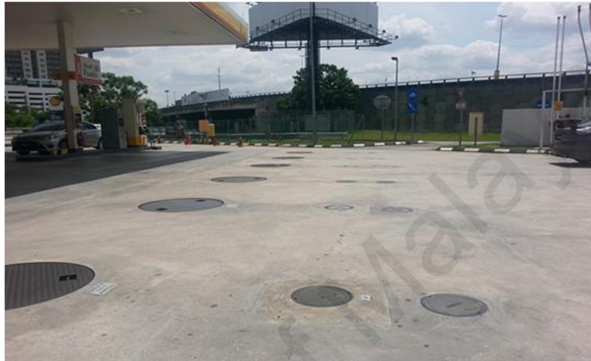
Figure 4.3 Underground storage tanks of hydrocarbon products
