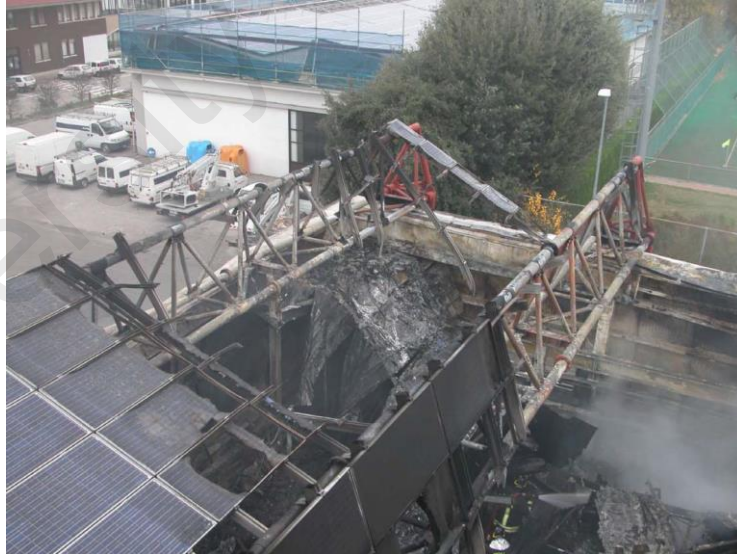
Figure 2.3: A 1000 sq. meter warehouse housing a roof-mounted PV system. (Ref. [25])
