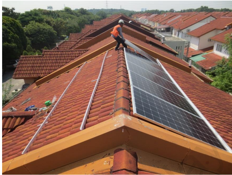
Figure 4.9: Worker arranging the Solar PV panel at residential rooftop
