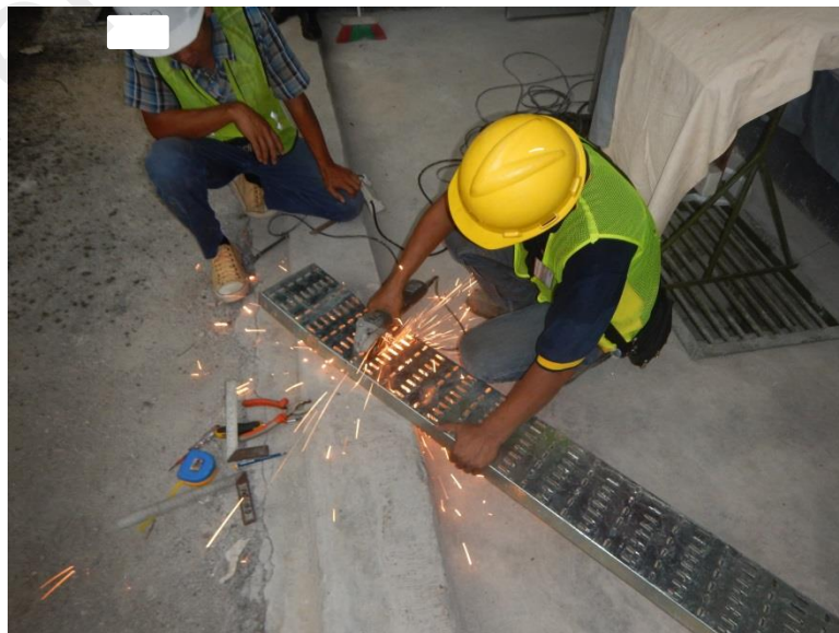
Figure 4.6: Worker was grinding the cable tray
