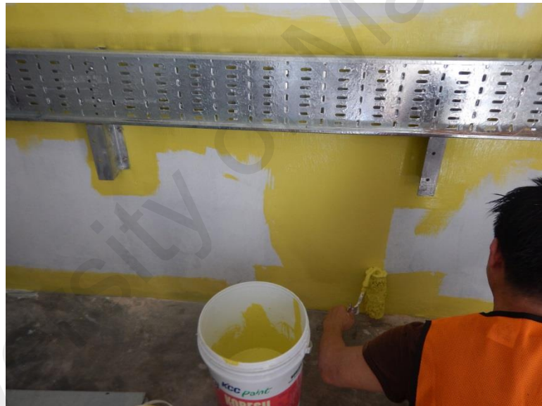
Figure 4.7: Worker was painting the inverter room
