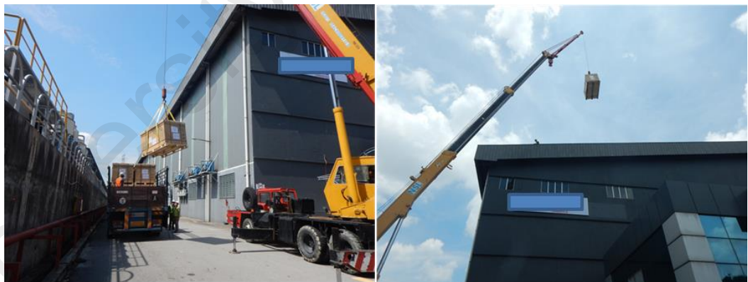
Figure 4.1: Loading and unloading of the Solar Panels at a Commercial building
