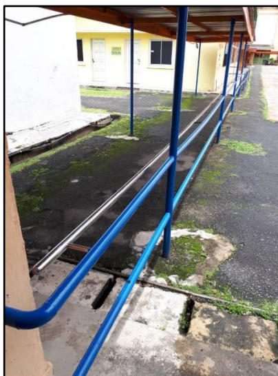
Figure 4.14: Safety hand rails at route to canteen.
