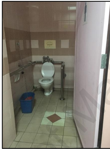
Figure 4.10: Toilet condition at School A.
