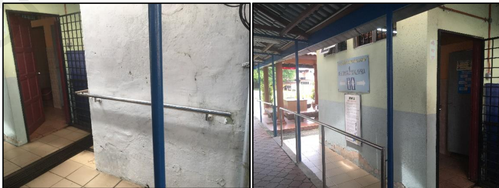
Figure 4.13: Safety hand rails at route to toilet.
