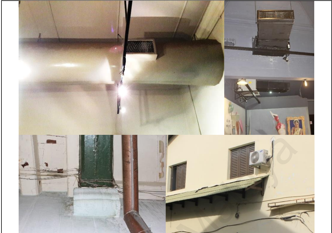
Figure 5.2: Inappropriate interventions made in regard to building services at the case studies
