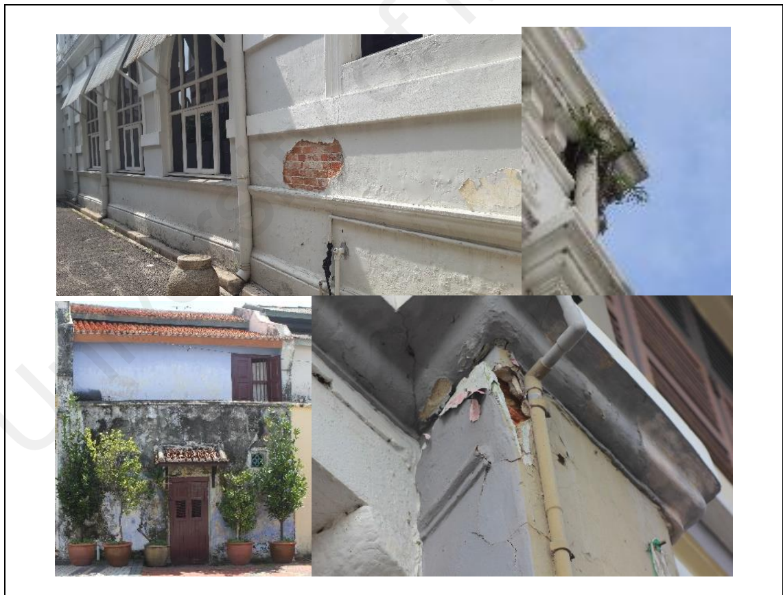
Figure 5.3: Peeling of paint finishes, unwanted biological growth, faded and mouldy surfaces and crumbling plastering work at the case studies
