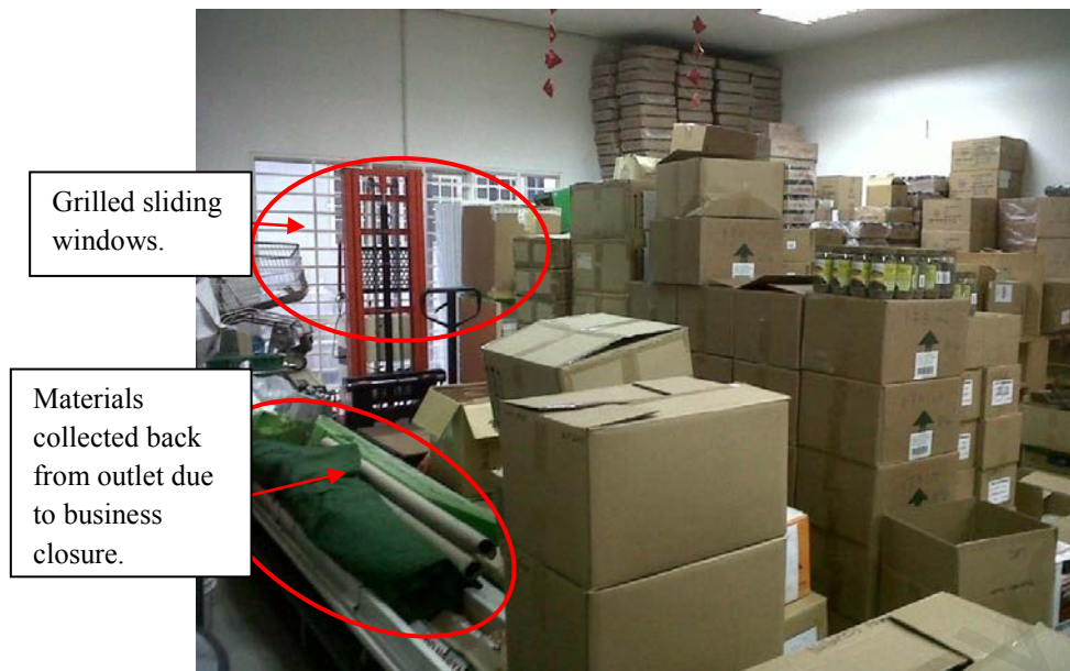
Figure 4.22: Blockage on another potential exit at the back of warehouse
