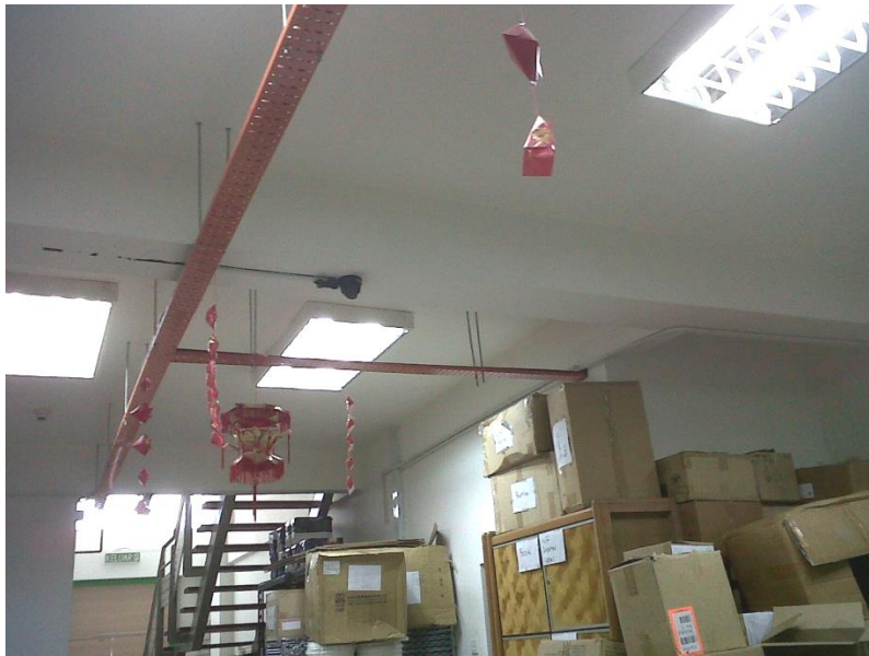
Figure 4.16: Placement of boxes which cluttered and disorganized
