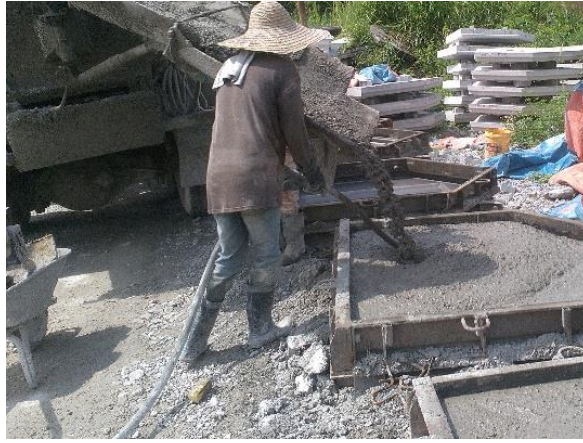
Figure 4.3: A poker vibrator use at fresh concrete
