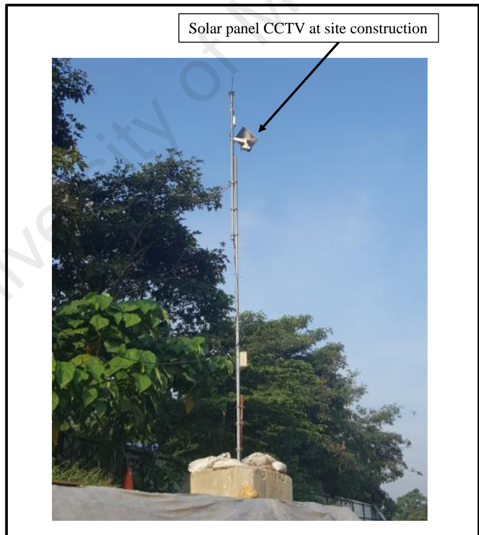
Figure 4.10: Solar Panel CCTV
