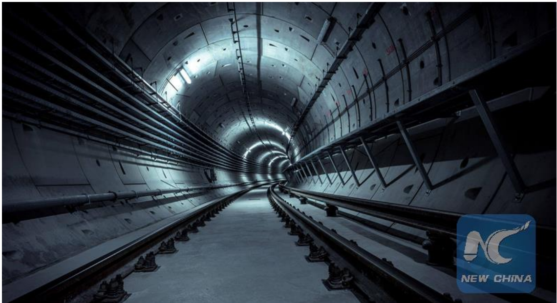
Figure 1.1: Sample of utility tunnel, ( http://www.xinhuanet.com )
