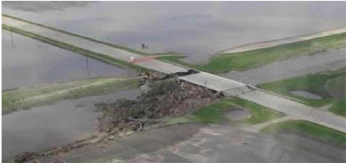
**Figure 1.3: A bridge failure in Wild River, Minnesota case caused by the interrelated action of scour and debris accumulation against the structure. (Ettema et al., 2006)**
