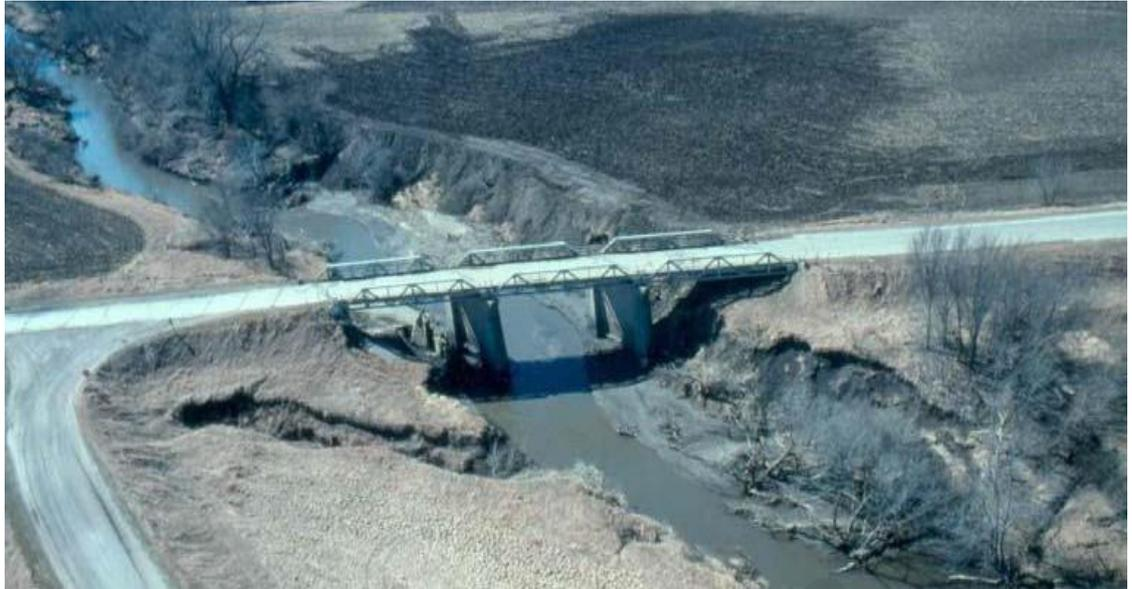
Figure 1.1: The Willow Creek bridge failure, where the bed elevation was lowered due to erosion. (Ettema et al., 2006)
