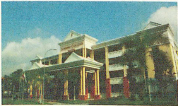
Kolej Sunway Johor Bahru
