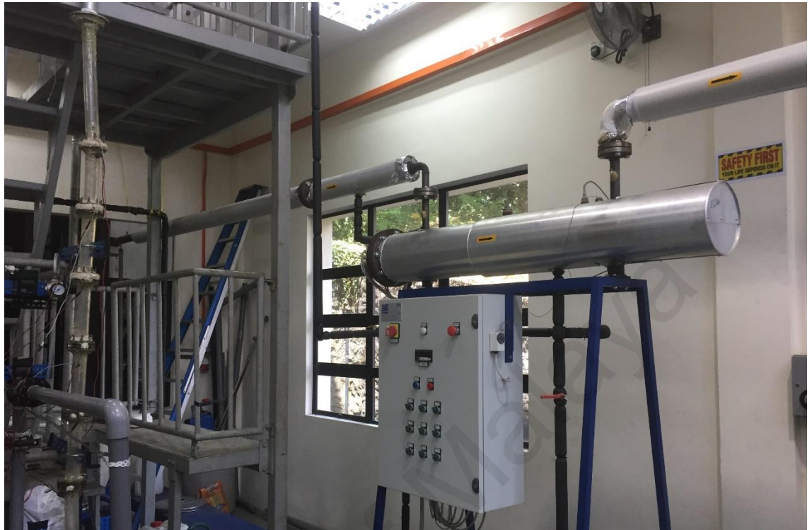
Figure 3.4: Superheater installed along the steam pipeline
