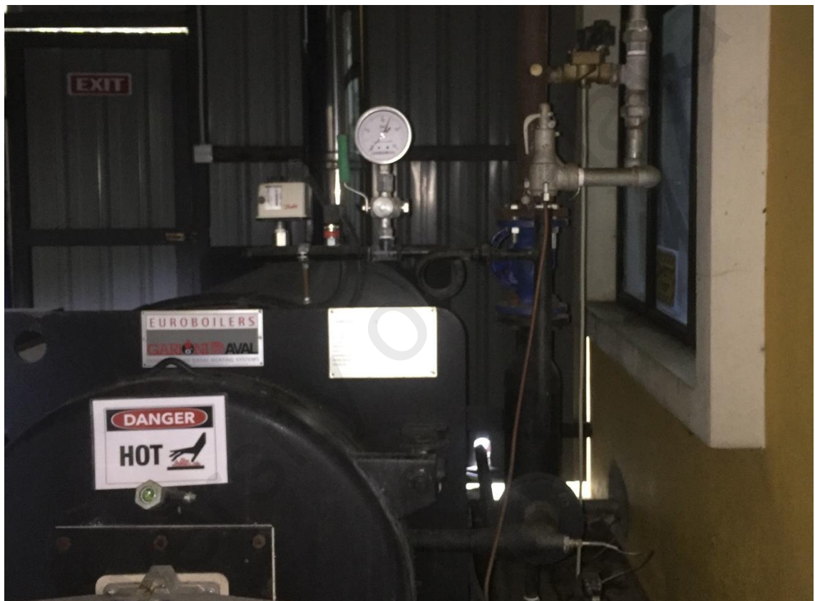
Figure 3.3: Pressure gauge, P_1 connected at boiler
