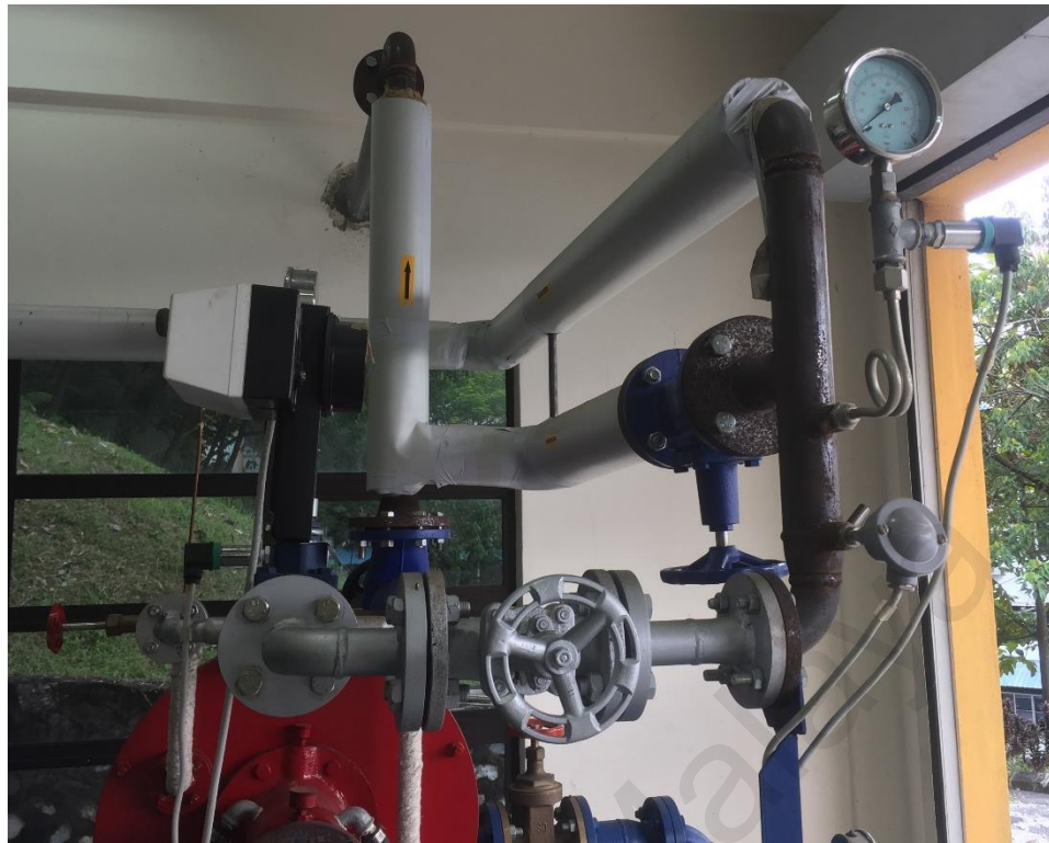
Figure 3.5: Pressure gauge, P_2 connected at turbine
