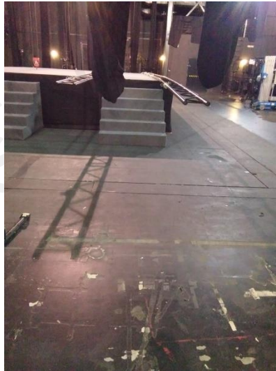
Figure 4.11: Protruding beams during stage set up at Pentas 1, Kuala Lumpur Performing Arts Centre, KLPAC
