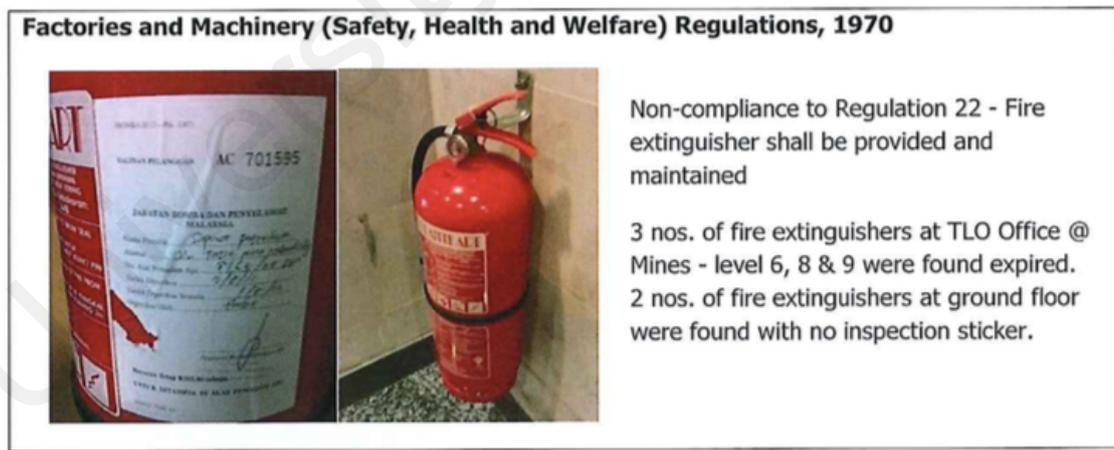
**Figure 4.1 Fire Extinguisher expired date of inspection**
