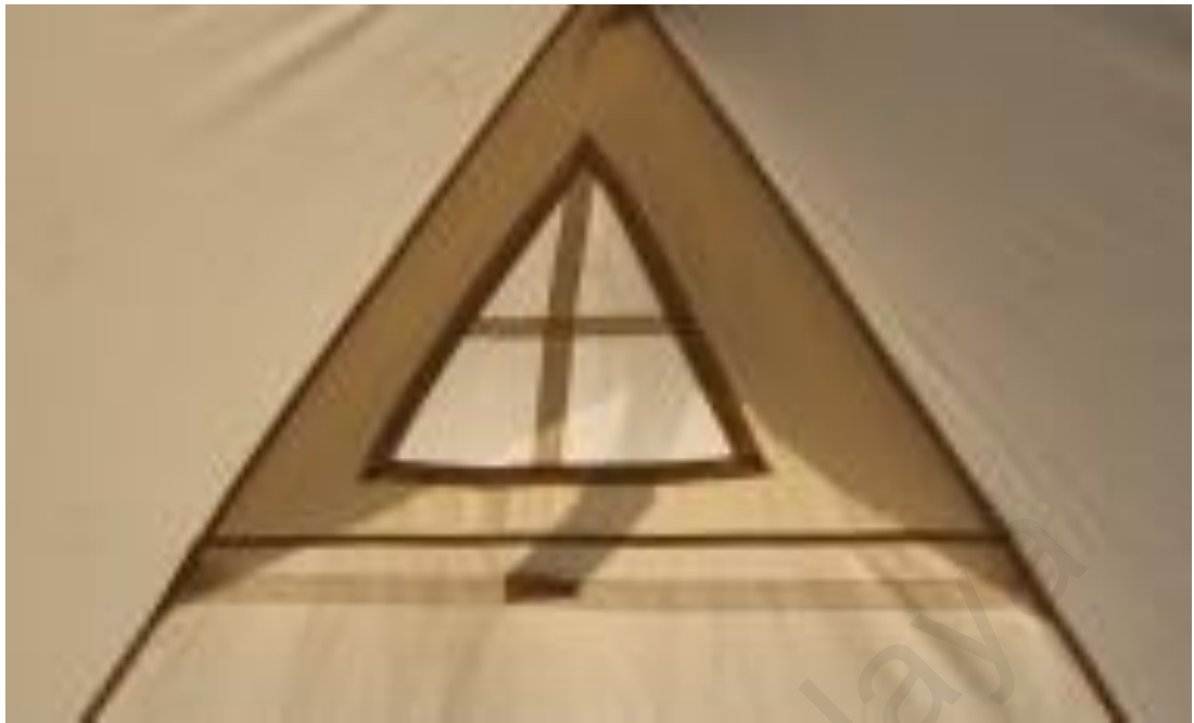
Figure 2.16: Interior View of Vent Openings for UNHCR Family Tent
