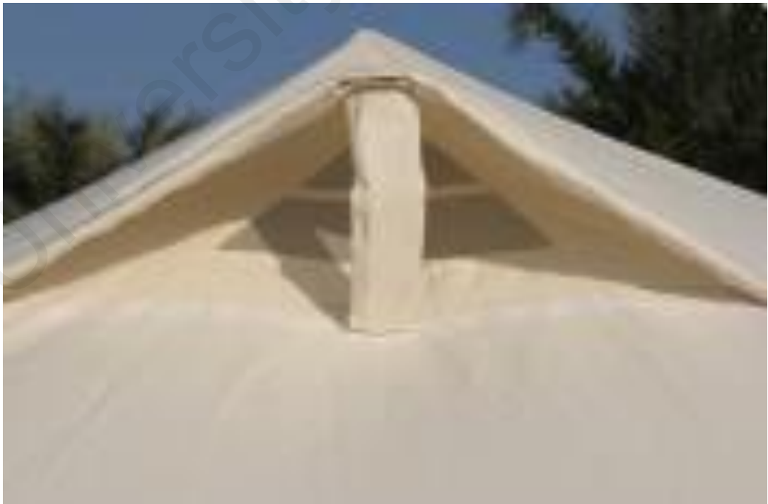
Figure 2.15: Exterior View of Vent Openings for UNHCR Family Tent
