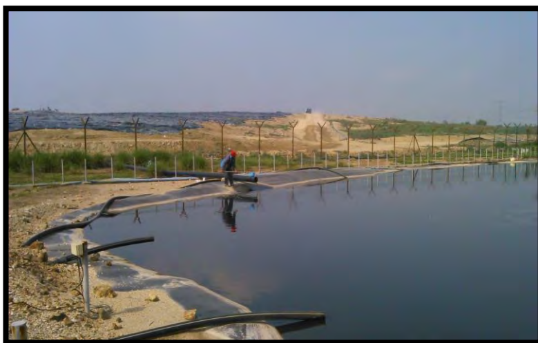
Plate 3.1 Pond collecting leachate in Jeram Sanitary Landfill
