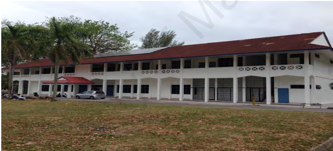
Figure 1.3. Image of silicon based solar cell setup: location archive building at Penang Free School, Penang, Malaysia.
