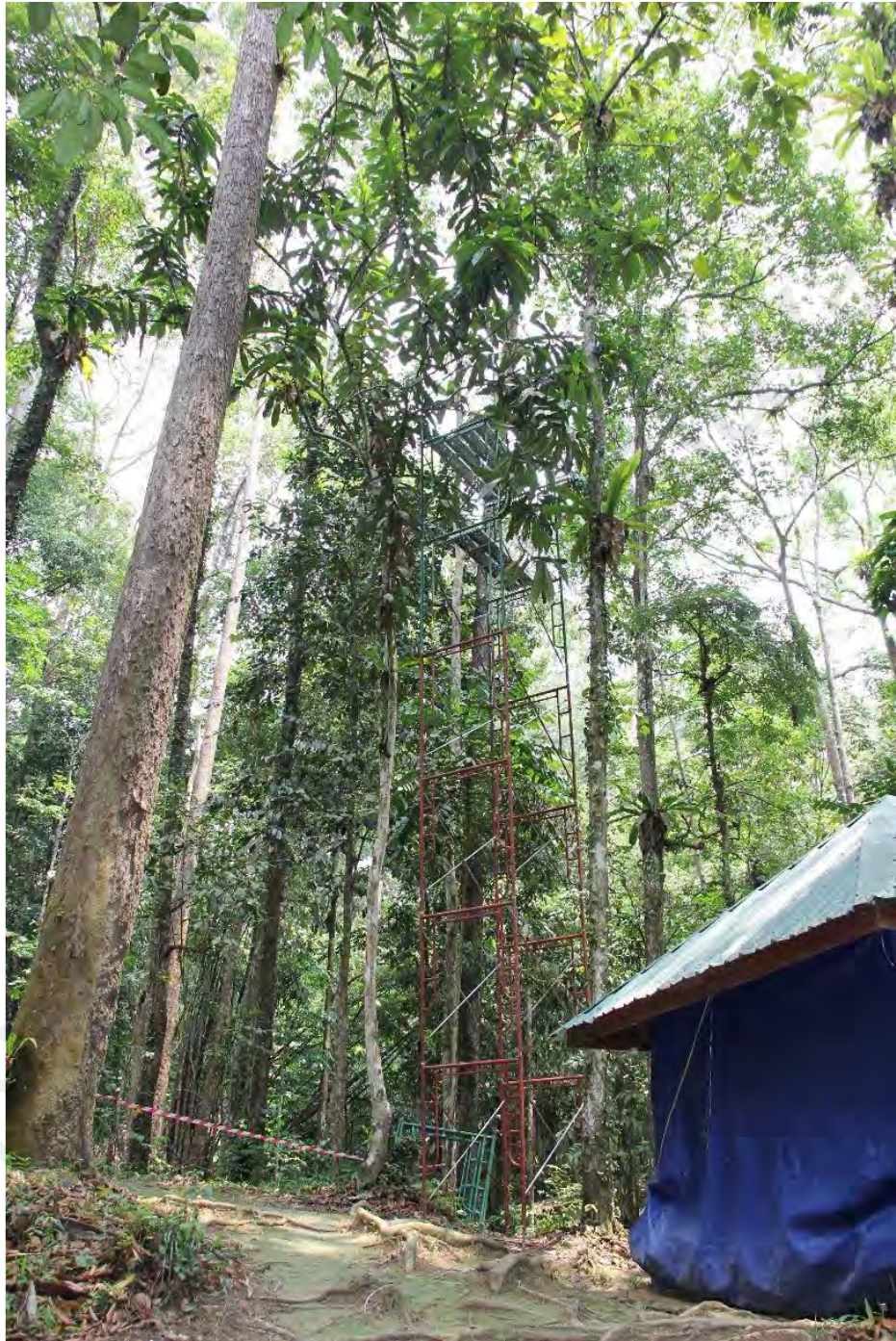
Figure 3.2: Scaffolding erected under Vatica yeechongii
