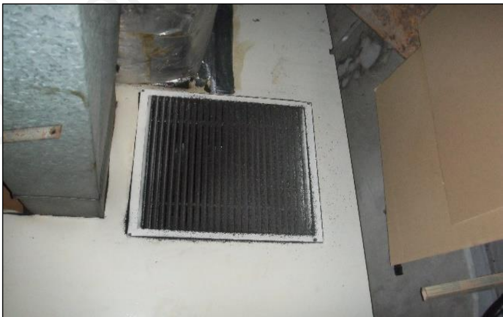
Figure 24 : Dusty fresh air intake grilles in one of Hospital A AHU.
