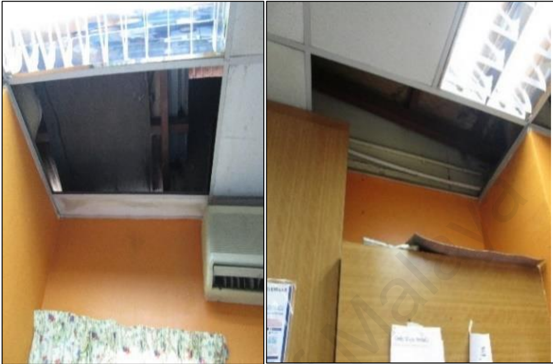
Figure 6 : Endoscopy Room with removed ceiling panel.
