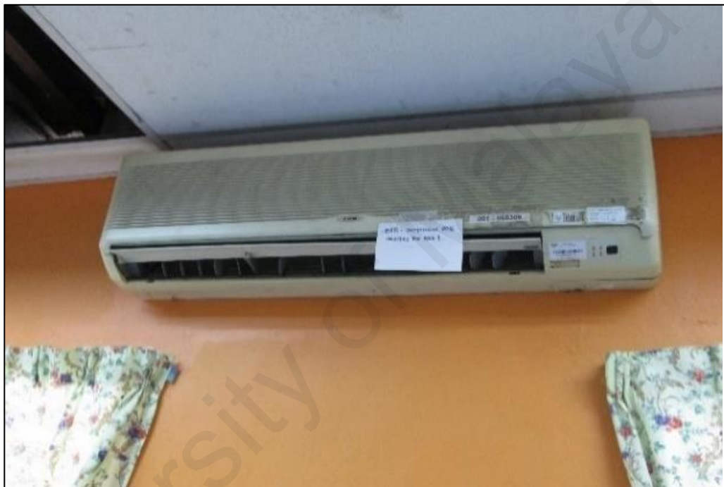
Figure 4 : Hospital A Endoscopy Room with malfunction air conditioning split unit.
