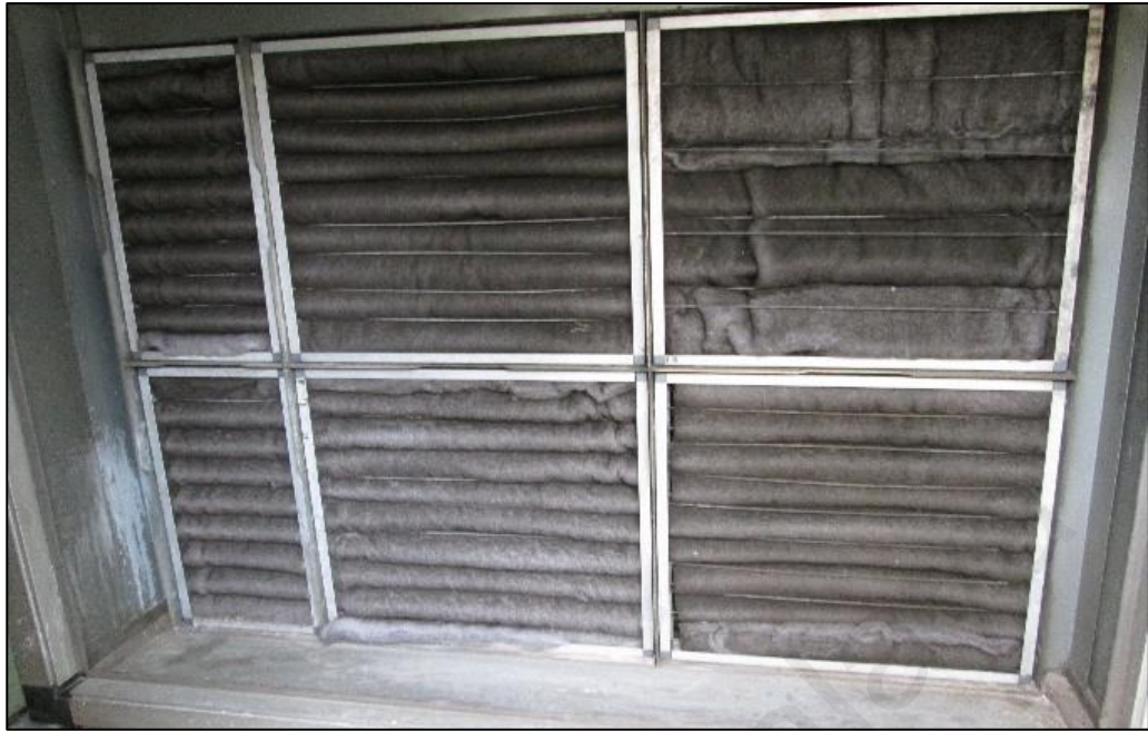
Figure 32 : Dirty pre-filters with accumulated dust.
