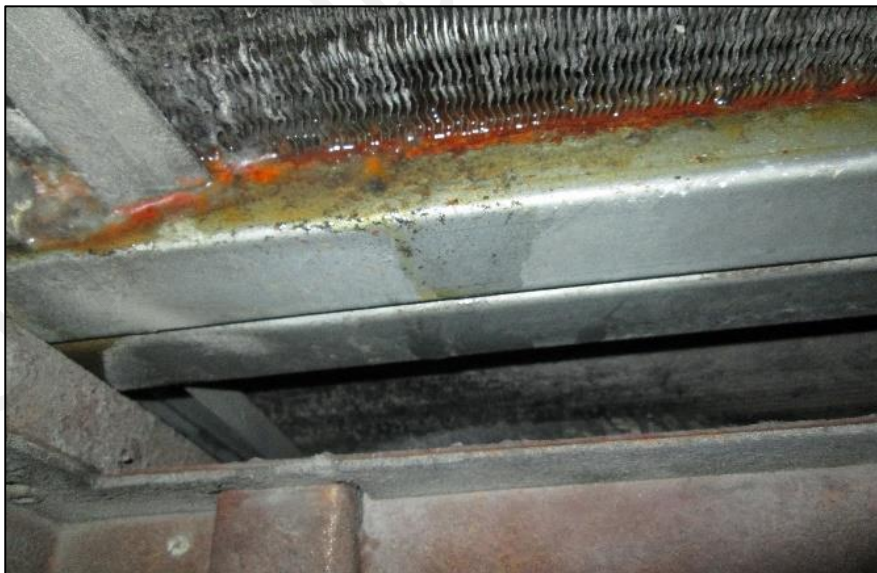
Figure 31 : Slime formation at cooling coils fin area (c).
