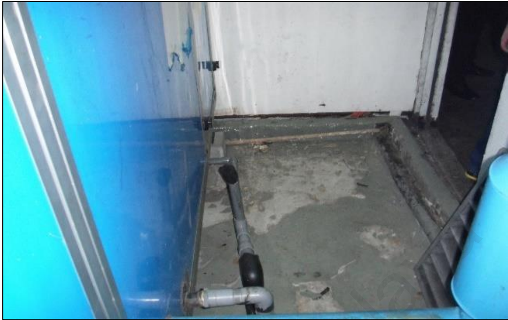
Figure 23 : Water ponding and leakage in one of Hospital A AHU.
