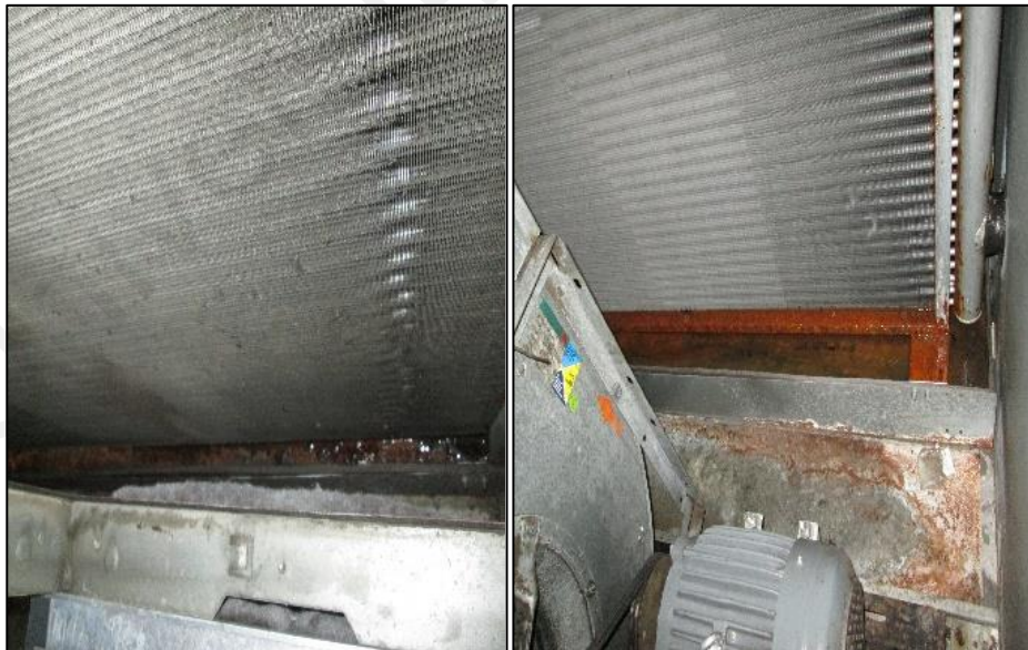
Figure 33 : Stagnant water and rusty drain pan in one of Hospital B AHU.
