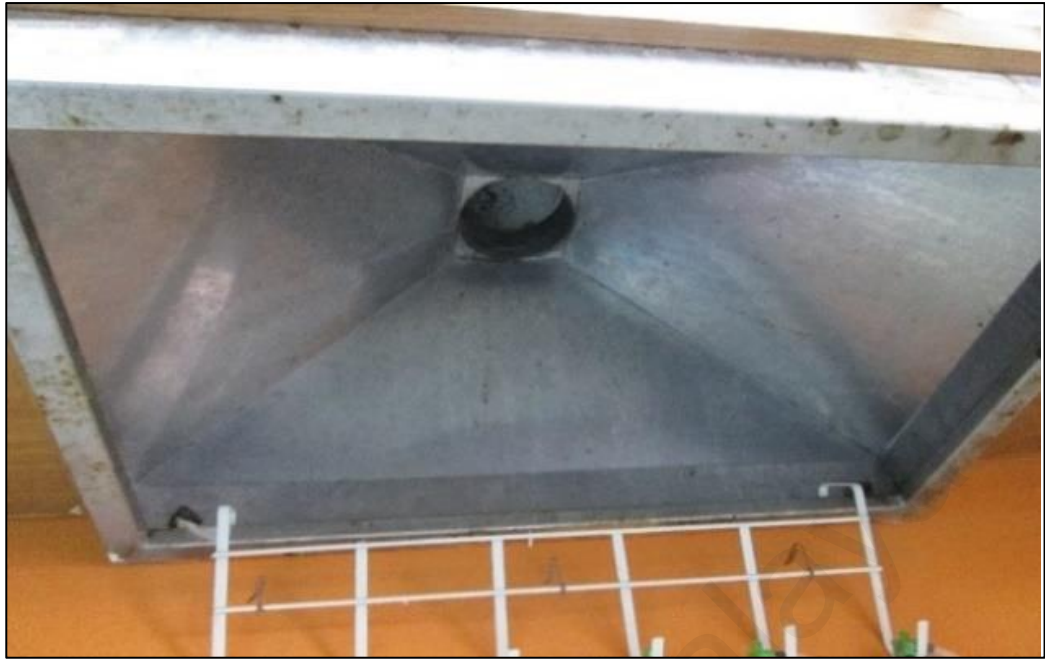
Figure 9 : Hospital C Endoscopy Room with malfunctioning fume hood.
