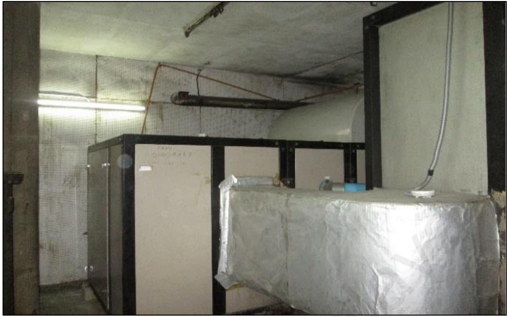
Figure 26 : One of AHU room condition in Hospital C.
