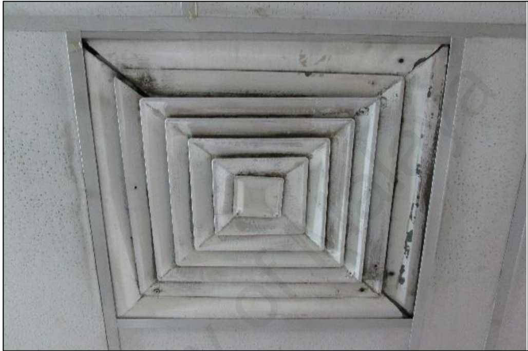
Figure 16 : Example of dusty supply diffusers.
