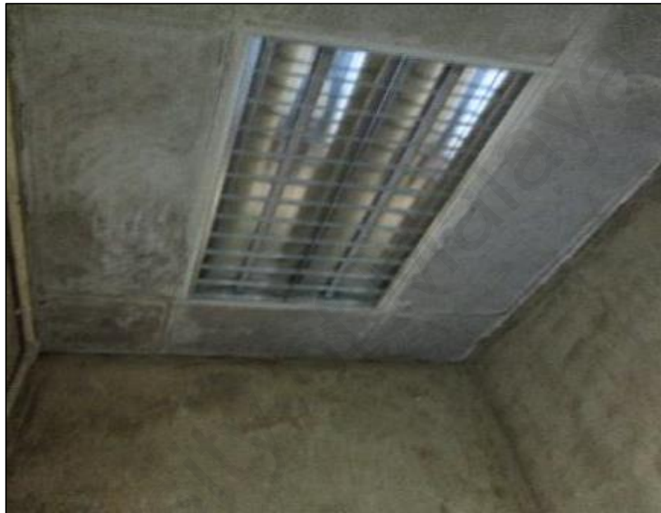
Figure 19 : Severe mold growth at Hospital A Autopsy Room (a)
