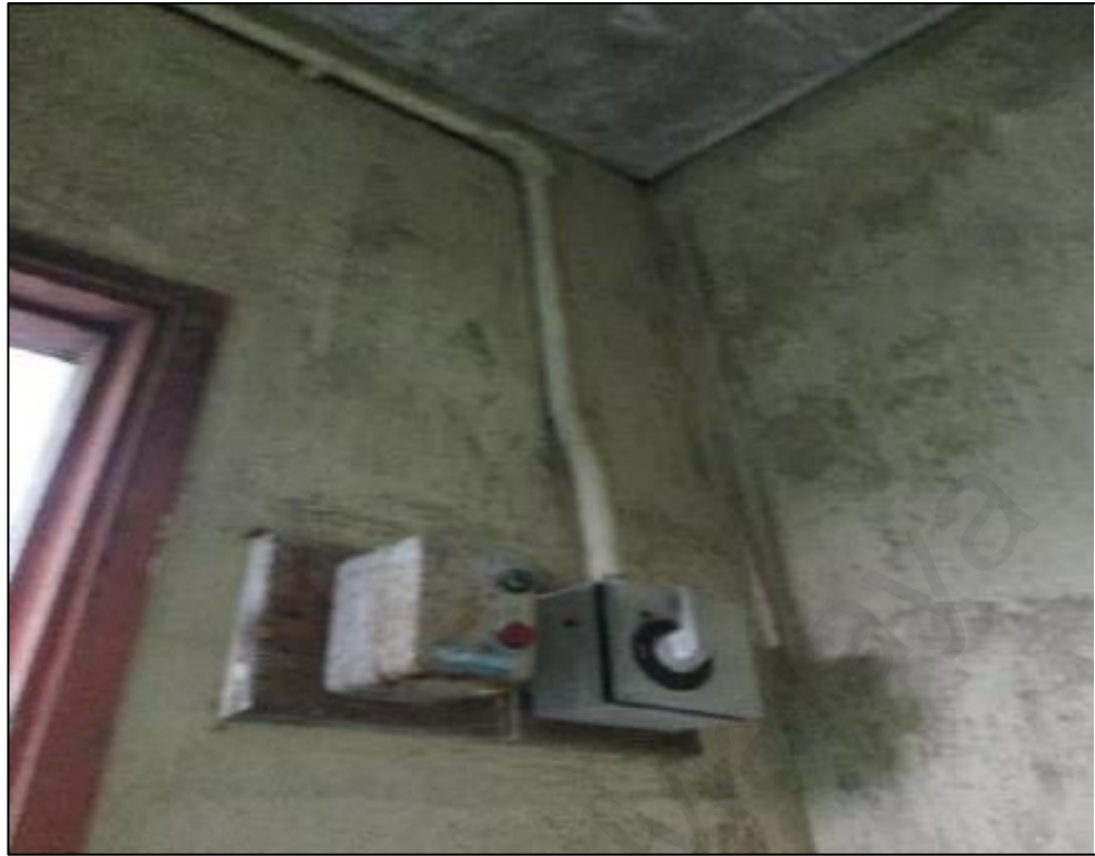
Figure 20 : Severe mold growth at Hospital A Autopsy Room (b)
