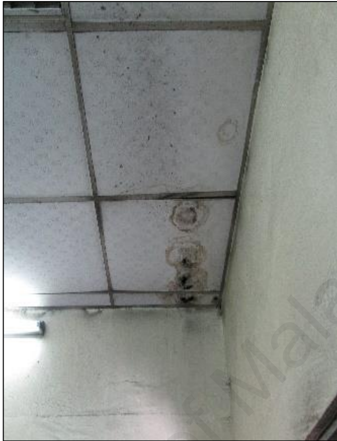
Figure 35 : Water stains with suspected water leakage at one of Hospital B AHU ceiling.
