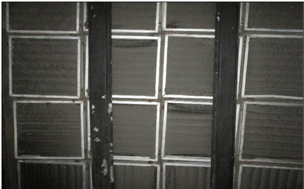
Figure 27 : Congested and dirty pre-filters in one of Hospital C AHU.
