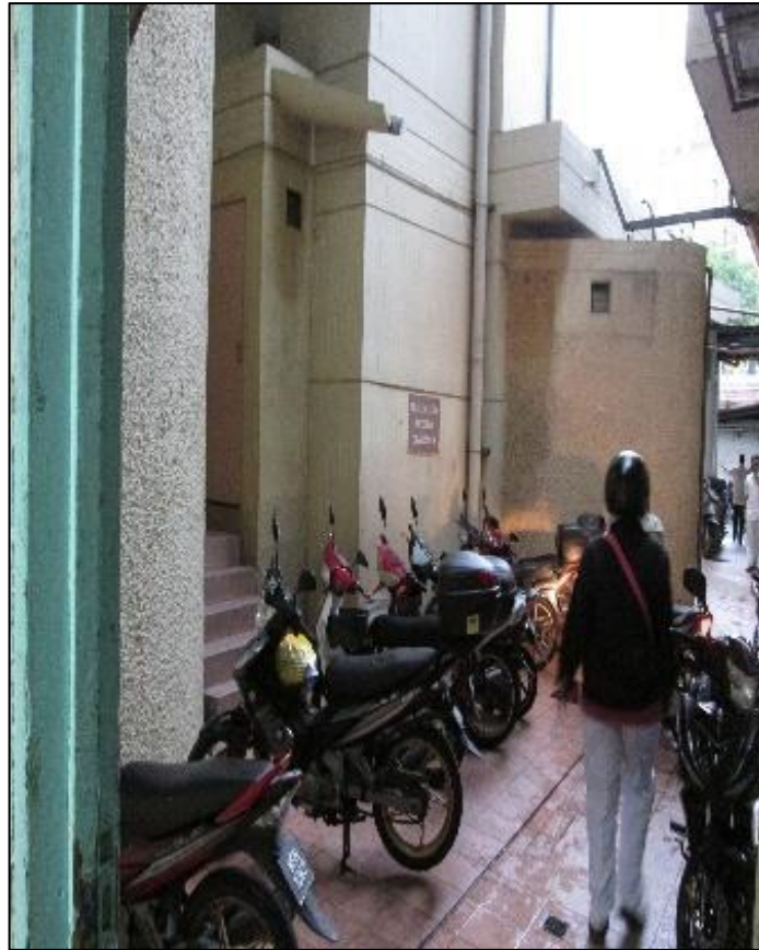
Figure 25 : Fresh air intake that facing outside motorcycle parking lot at Hospital A.
