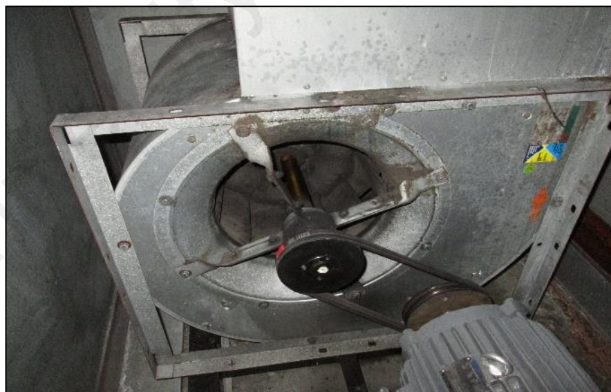
Figure 36 : Dusty blower fans.
