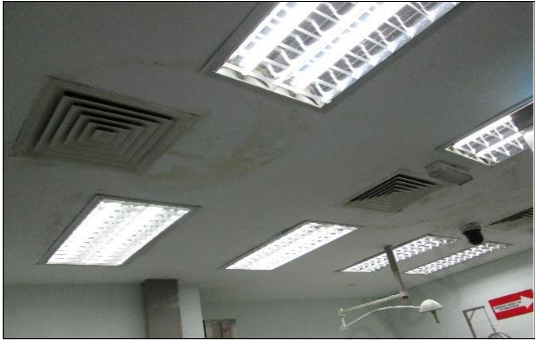
Figure 21 : Mold growth and water stains at Hospital B Autopsy Room.
