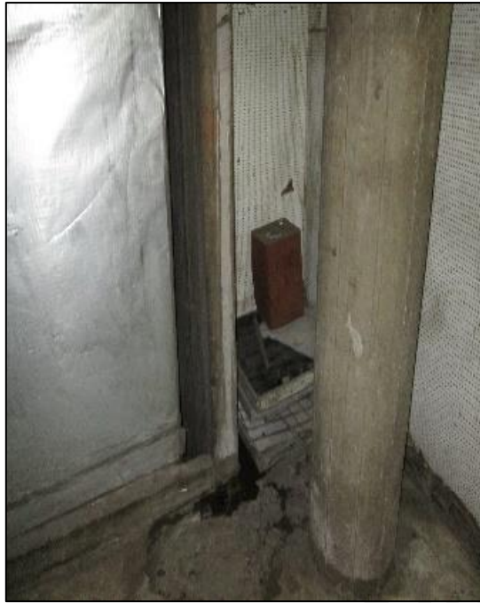
Figure 30 : Unused items and consumable parts left unattended (c).
