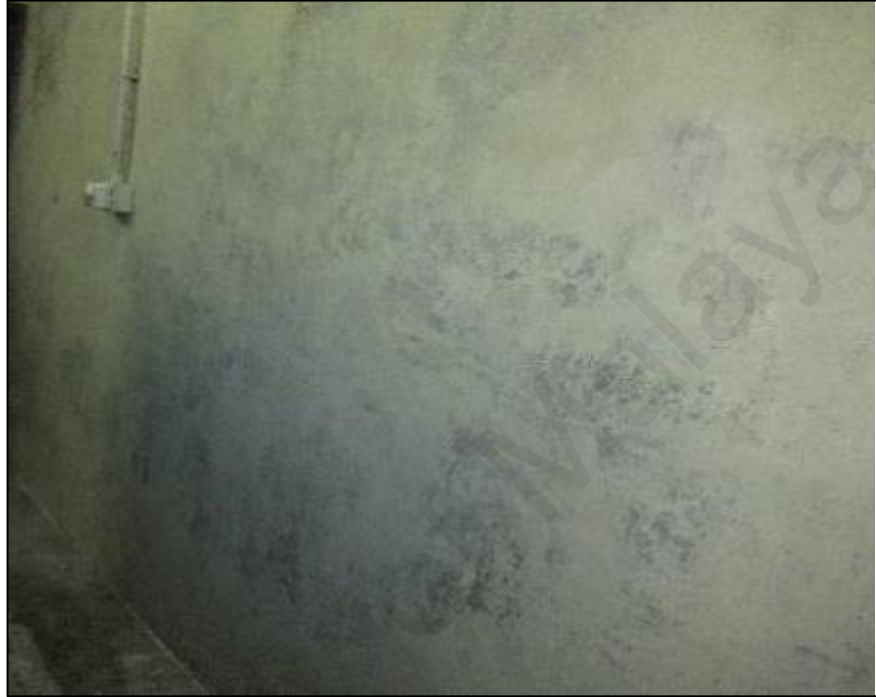
Figure 34 : Mold stains in one of Hospital B AHU wall and ceiling.
