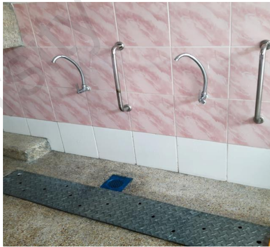
Figure 3.9: Ablution Workstation at Surau Al-Hidayah, PLPP Bangi
